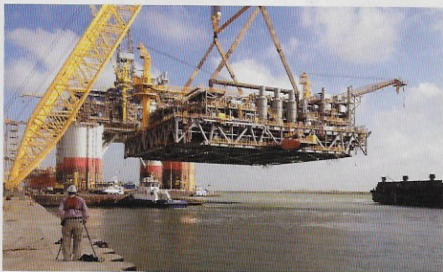
The single-lift of the topsides was required to achieve LLOG's accelerated project schedule.
